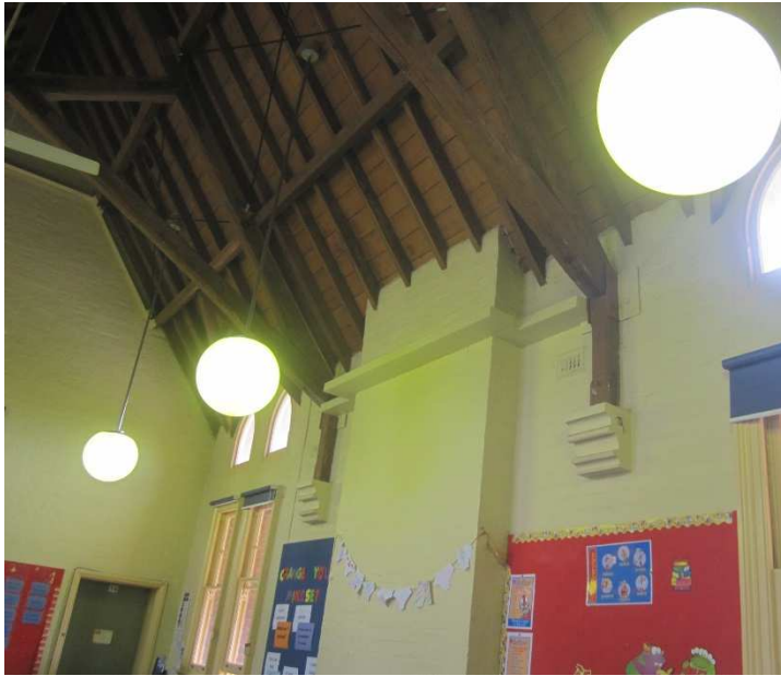
Figure 7 – Shows steel channel beam between roof trusses for chimney.
