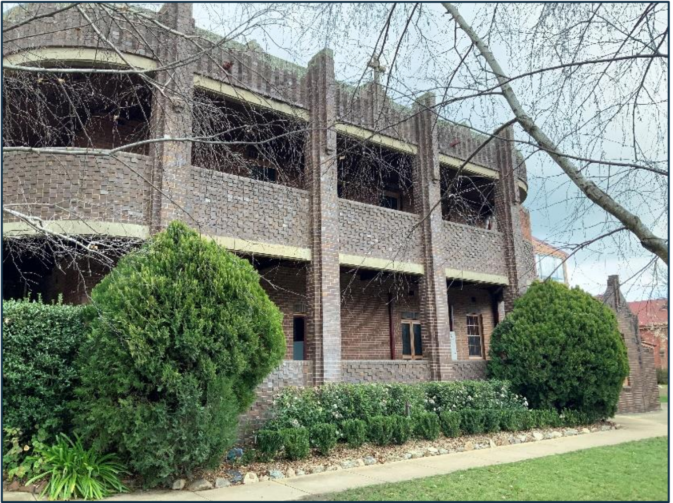
FIGURE 2 - REAR OF THE EXISTING ADMINISTRATION BUILDING
