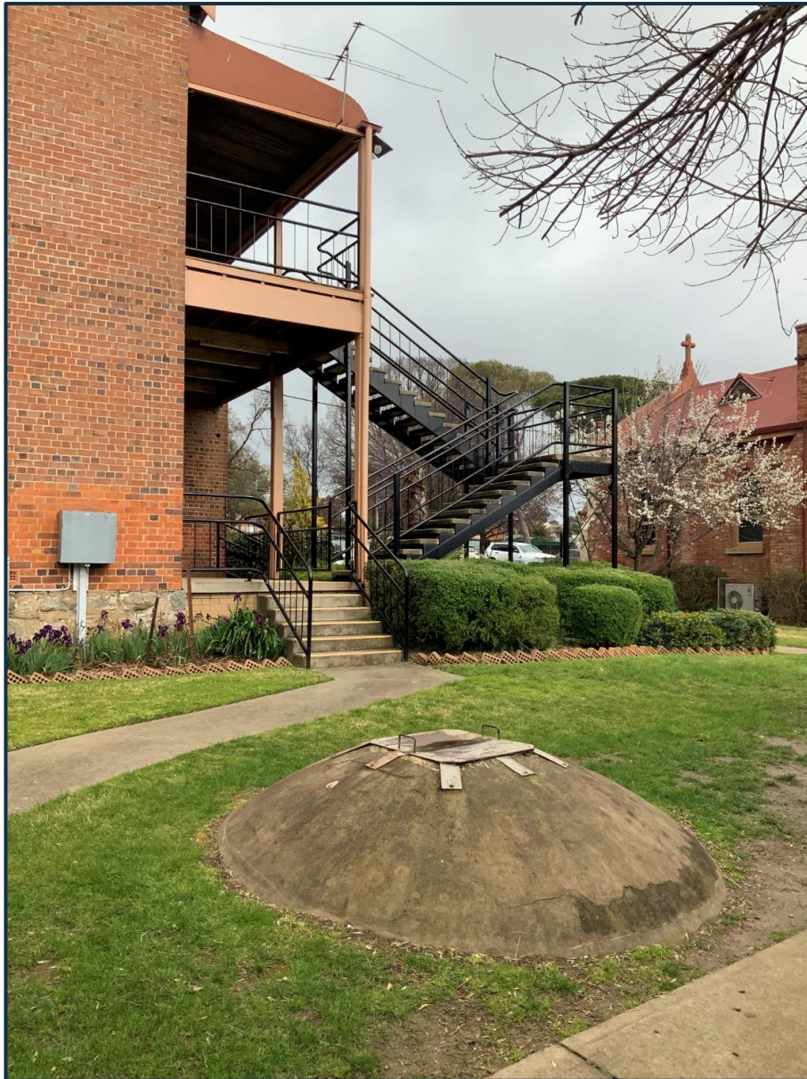
FIGURE 23 - CONCRETE DOME AT THE NATURAL GROUND LEVEL (REAR OF BUILDING)
