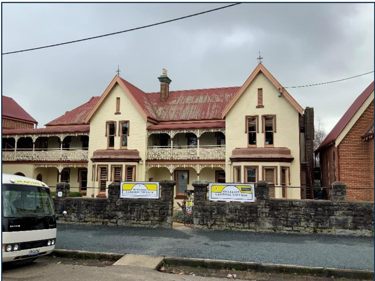
FIGURE 1 - FRONT OF THE EXISTING ADMINISTRATION BUILDING
