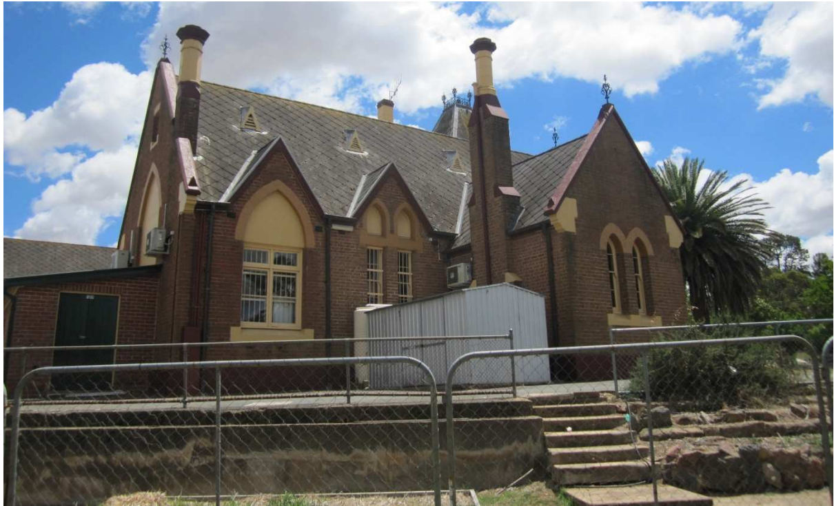
Figure 3 – South-East Elevation – showing two tall chimneys, two gable walls and two gablets
