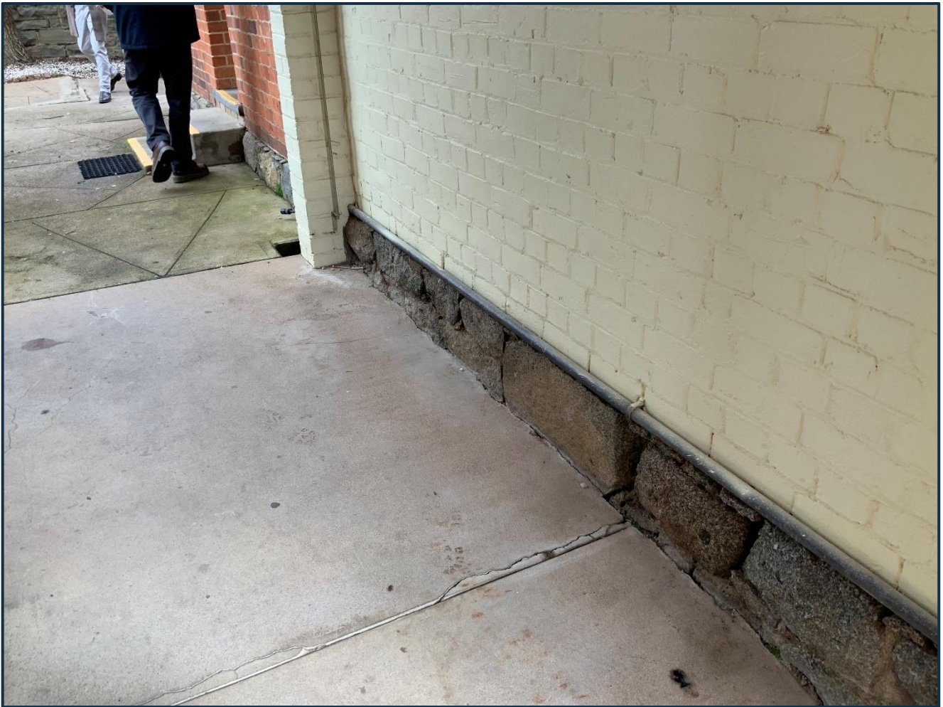
FIGURE 3 - SITE PHOTO OF THE EXISTING EXTERNAL PERIMETER BUILDING FOUNDATIONS
